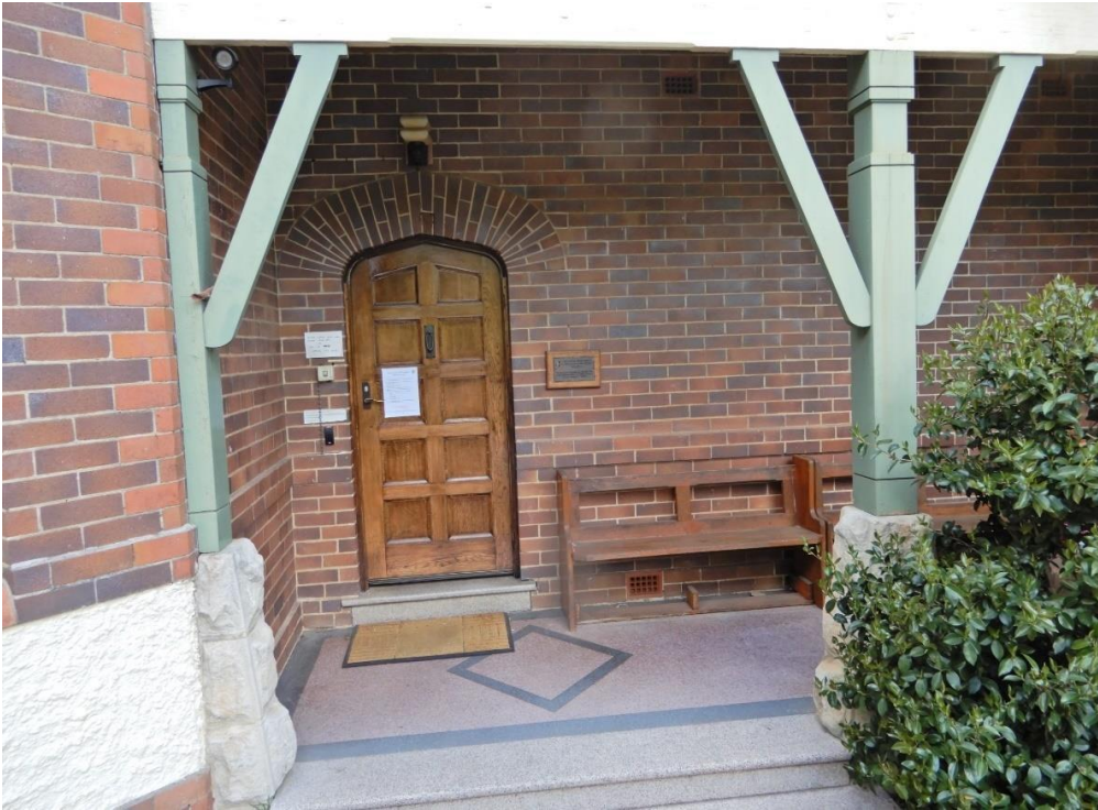
Figure 19: the front central recessed bay is a wall that was rebuilt in 1938, providing a new front door in Inter-war Old English (Tudor) style with an ogee arch. The terrazzo verandah floor is from 1938, but it appears that the verandah columns were reinstated over it.
