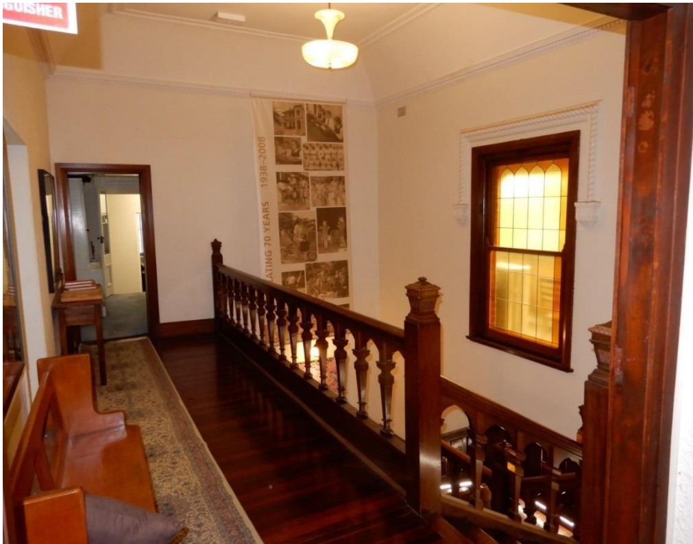
Figure 29 — the stair hall between the faceted bays and the amber-glass window are likely an Inter-War Old English style alteration within the house.
