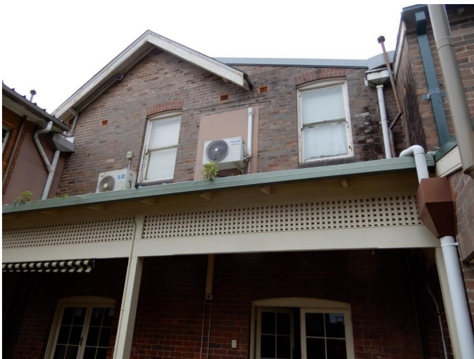
Figure 22 — the rear east-facing façade retains early brick work and windows at the first floor. The upper part of the gable may be an early extension, followed by the low-pitched valley on the right with much evidence of alteration, The 1960s former dormitory wing is glimpsed on the left.
