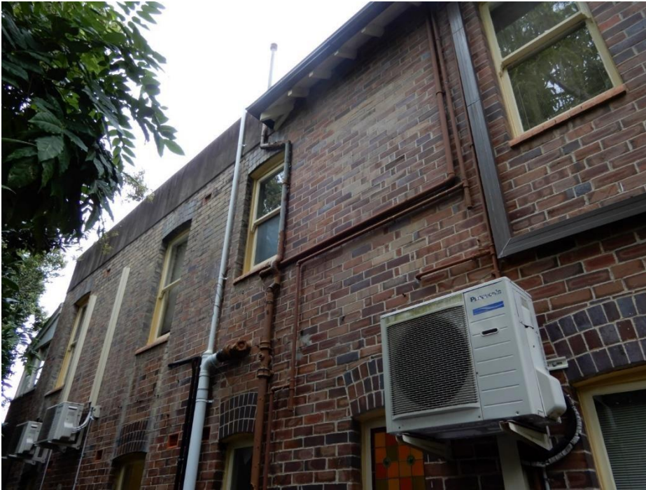
Figure 21 — the northern side wall of the building has a Federation character, although there are many signs of early alterations. The ground floor wall is likely original, and the first floor with its rendered parapet appears to be an early extension.
