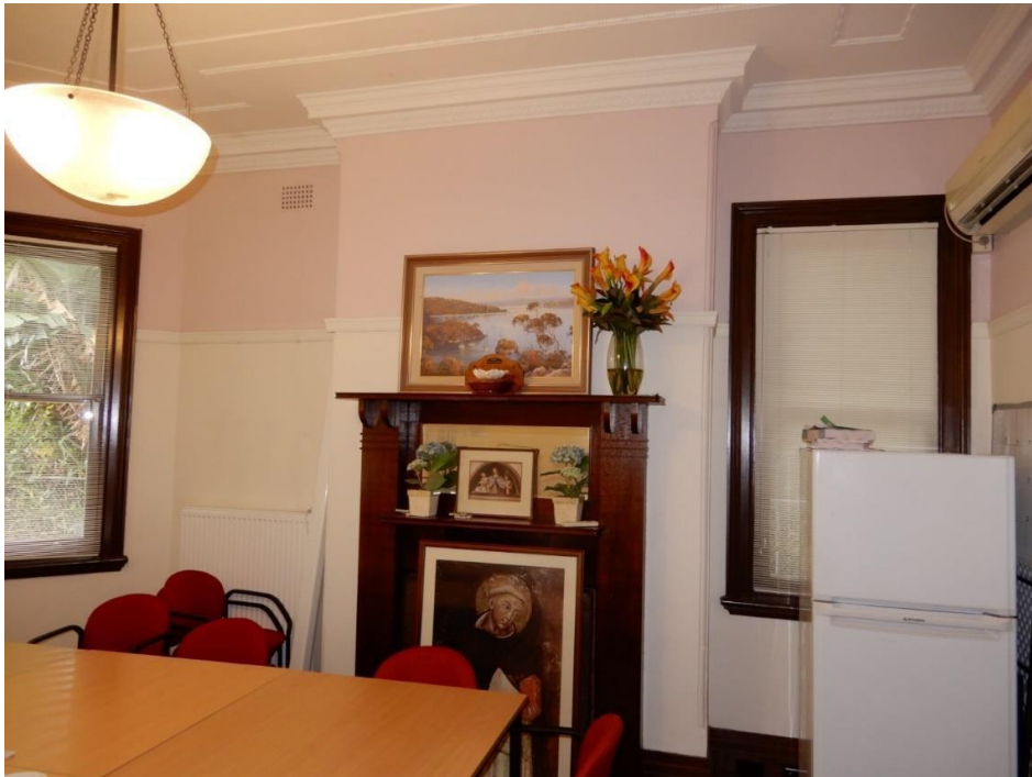
Figure 28: the ground-floor north-western room retains its likely original skirting, architraves and mantelpiece. The cornice appears to have been altered in the 1930s.
